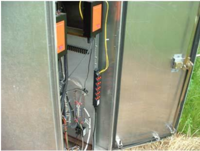
Above photo shows a GatorPatch installed in a typical traffic control cabinet. The blunt (pigtail) end of the cable is spliced to the main underground trunk cable
